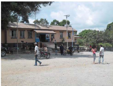
TANKORO POLICE STATION
