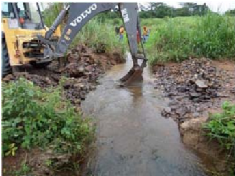
REPLACEMENT OF CULVERT TO LINK BUMPEH KOIDU TO JAIMA-NIMIKORO ROAD
