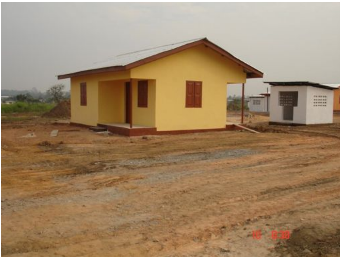
NEW HOUSE BUILT FOR TAMBA KAIFALA
