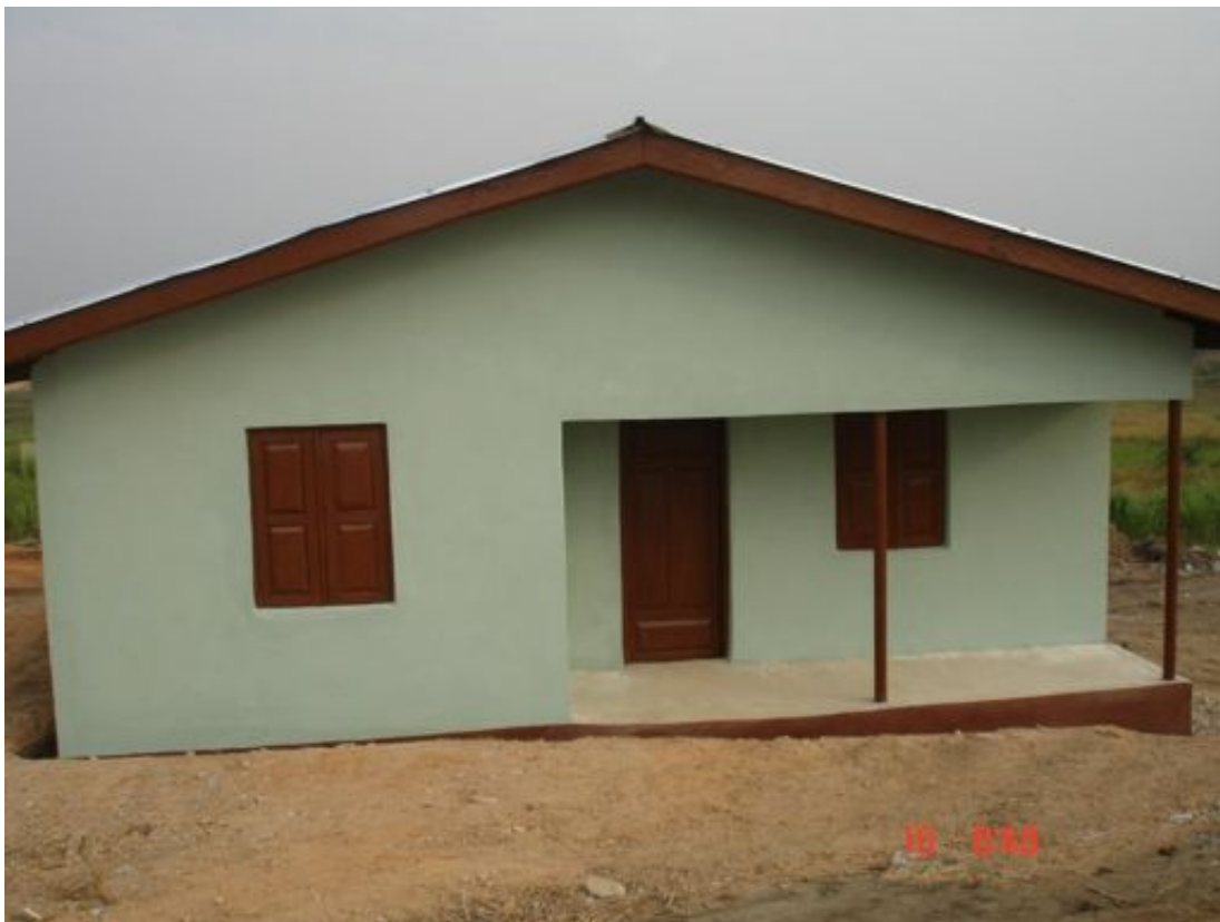
NEW HOUSE BUILT FOR KUMBA ISSAH
