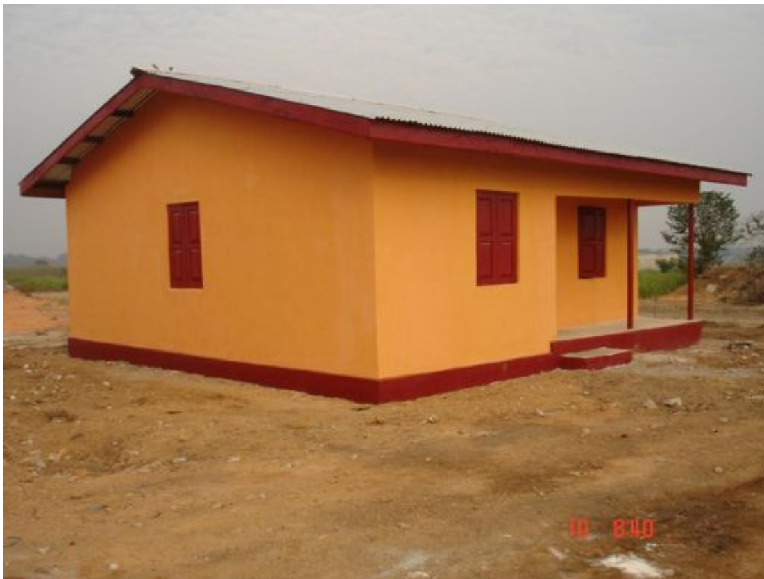
NEW HOUSE BUILT FOR KAI ALLIEU
