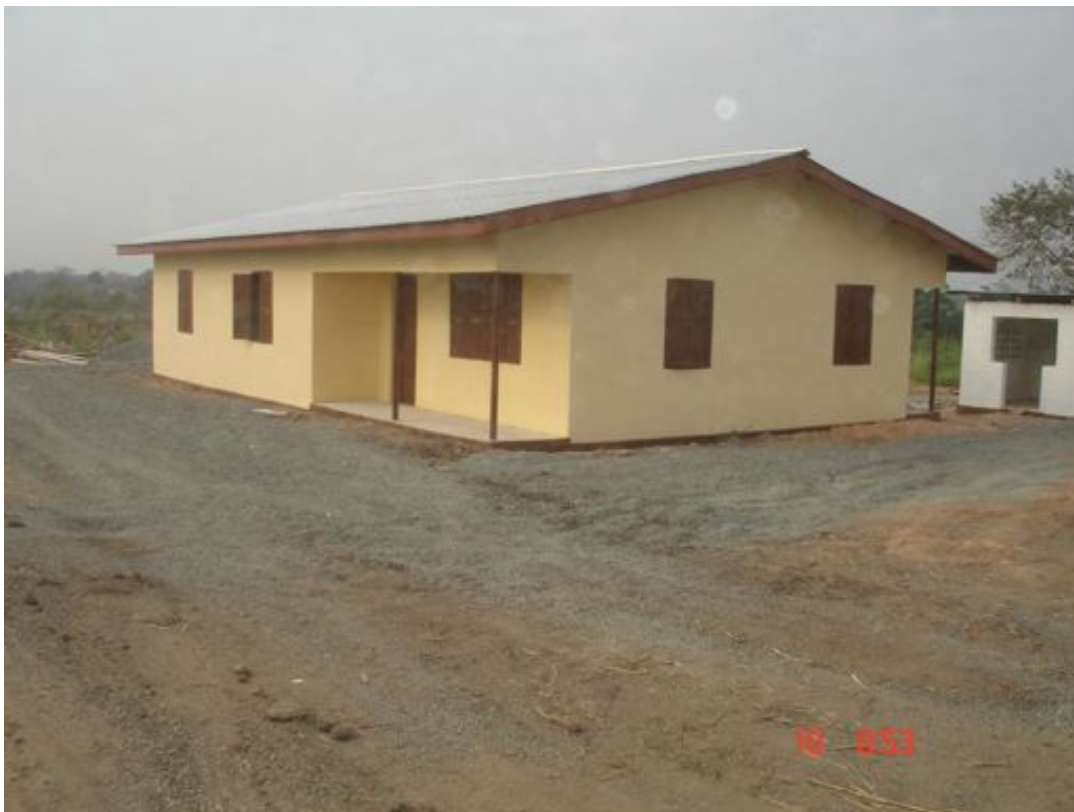
NEW HOUSE BUILT FOR SIA ALUSINE
